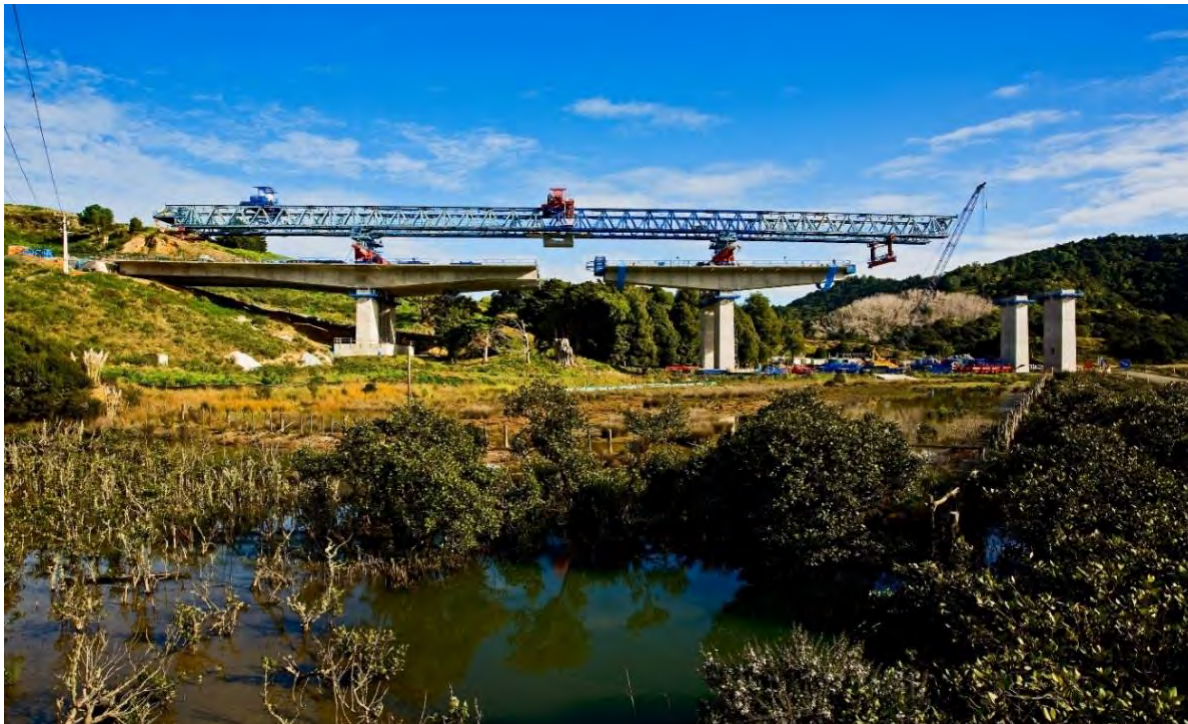
Figure 5-7: A launching gantry placing segmental box girder sections on the Waiwera Viaduct
